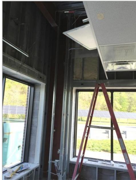
*Tear down of existing batts insulation and drywall can be labor intensive.*
