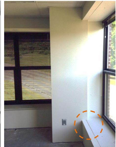
*Extended window frame over additional insulation thickness*
