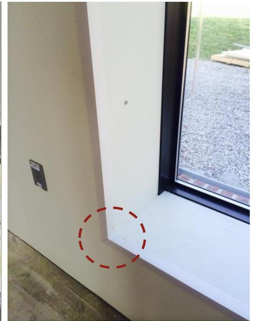
*Extended window frame over additional insulation thickness*
