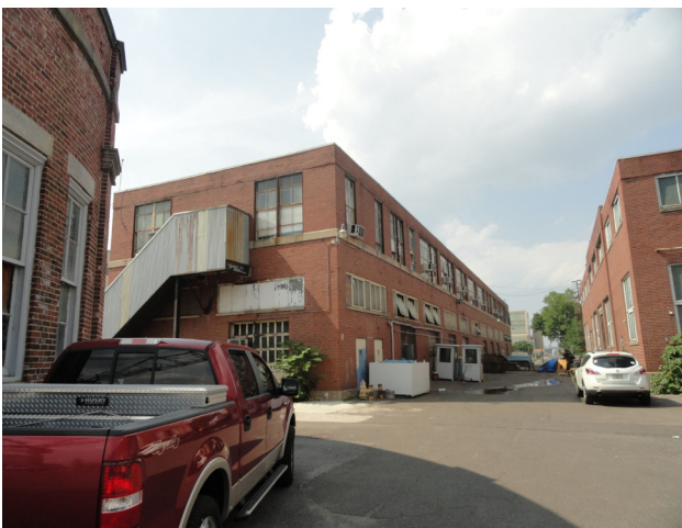
Philadelphia Navy Yard Building 669 during a site assessment. Source: EEB Hub
