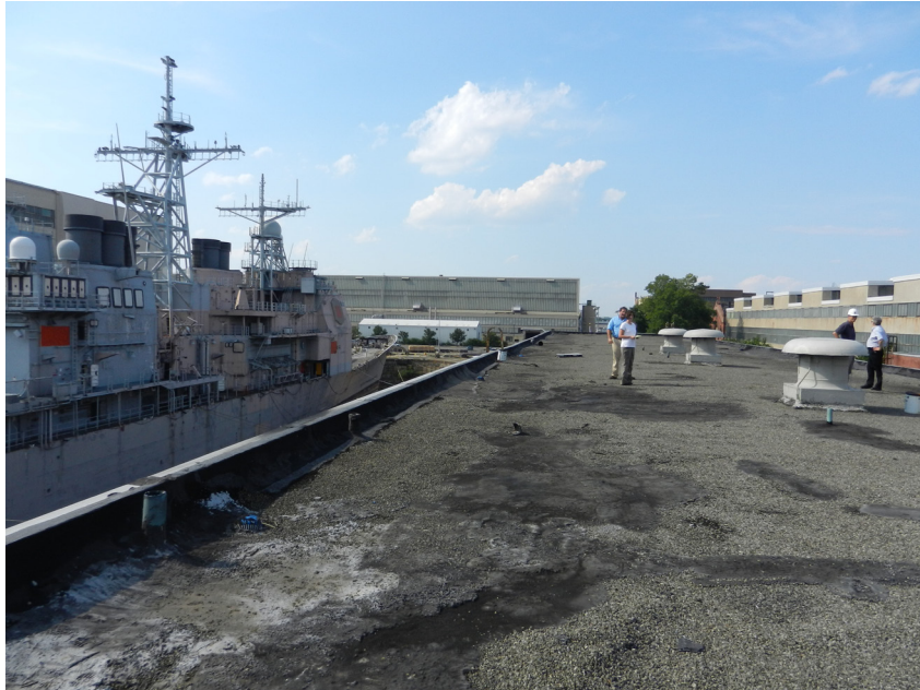
Philadelphia Navy Yard Building 669 from the roof during a site assessment. The adjacent dry dock is visible to the right.
