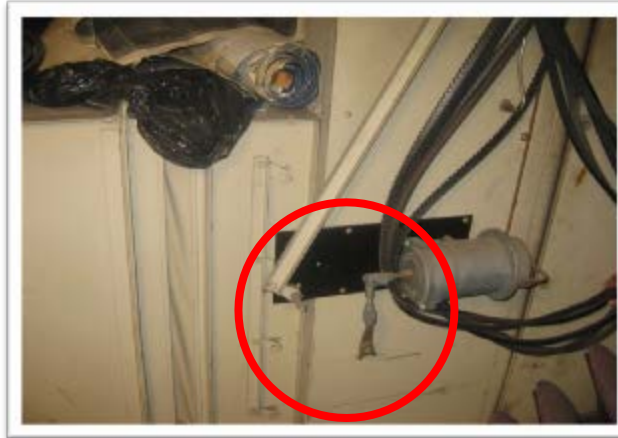
Disconnected Damper
