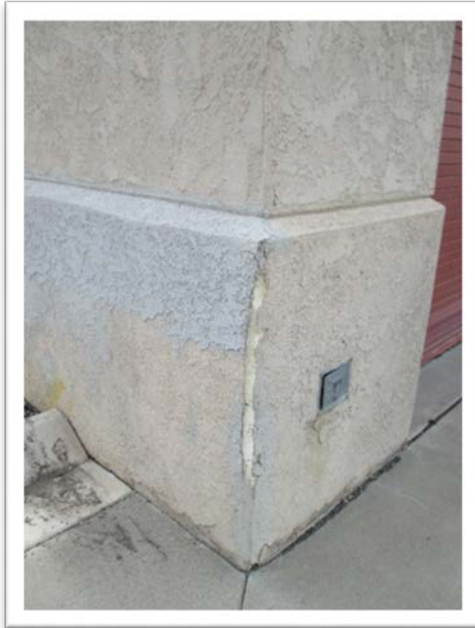
Cracked and deteriorated EIFS material, exposing insulation to elements
