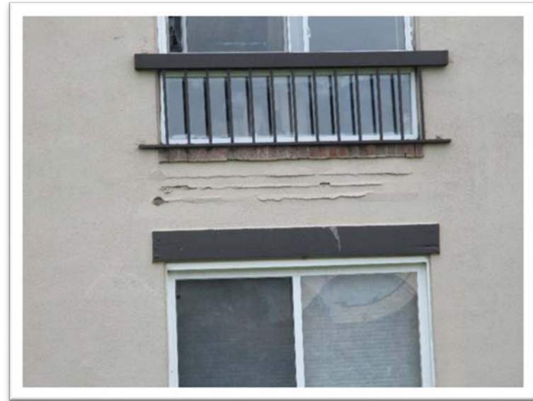
Damage to exterior material leading to potential water infiltration
