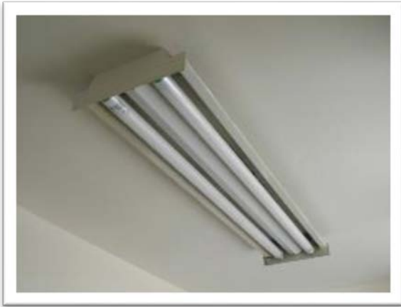
T-12 lighting should be switched out
