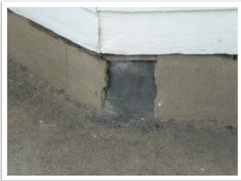
Cracks and penetrations in the foundation
