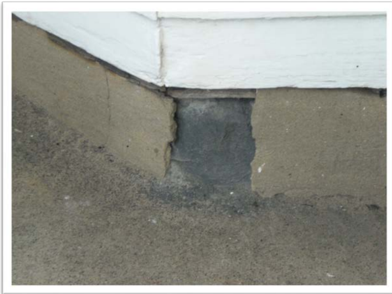
Cracks and penetrations in the foundation
