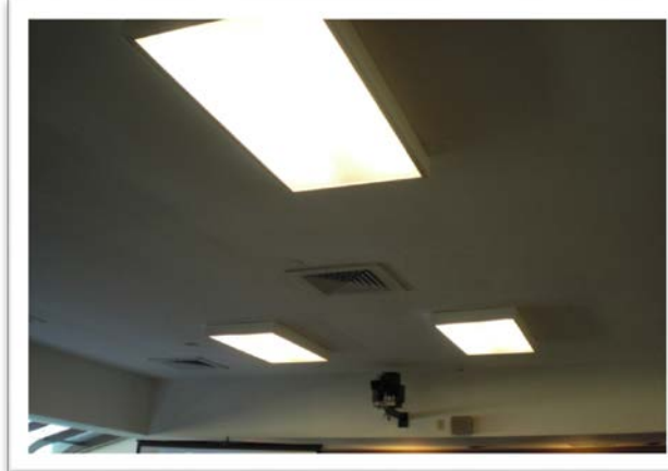
Convert magnetic ballasts to electronic
