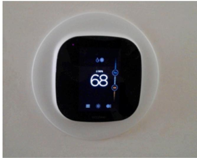
Figure 12: Ecobee3 Wi-Fi thermostat
