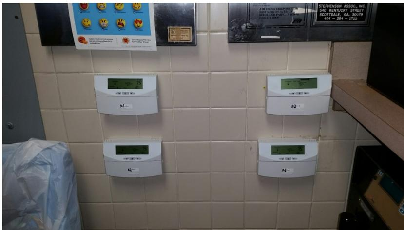
**Figure 8: Typical Honeywell based thermostat installation at JACE sites (remote temperature sensors are employed to obtain measurements in the controlled spaces)**
