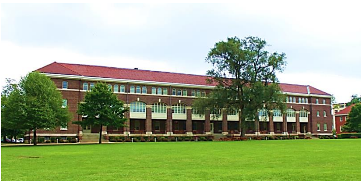
Building 101 located at The Navy Yard in Philadelphia
