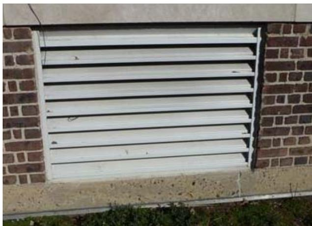
Figure 5.8 Outdoor air intake unmasked
