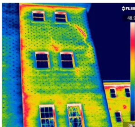
Figure 5.1 Heat loss through wall cracks
