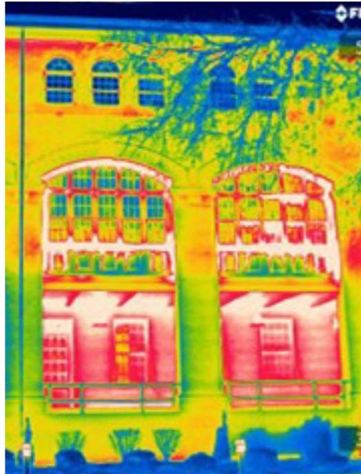
Figure 14. Heat loss through cracks in window frames
