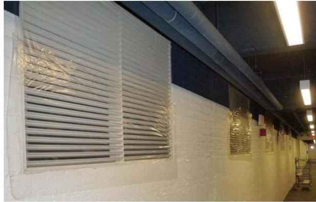
Figure 5.7 Fire control dampers initially sealed with self-adhering duct mask
