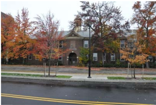
Figure 1: 661 Front (east) View
